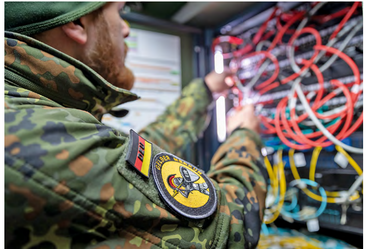
Bundeswehr IT exercise GELBER MERKUR 2023 – electronic monitoring of communication channels via cable
